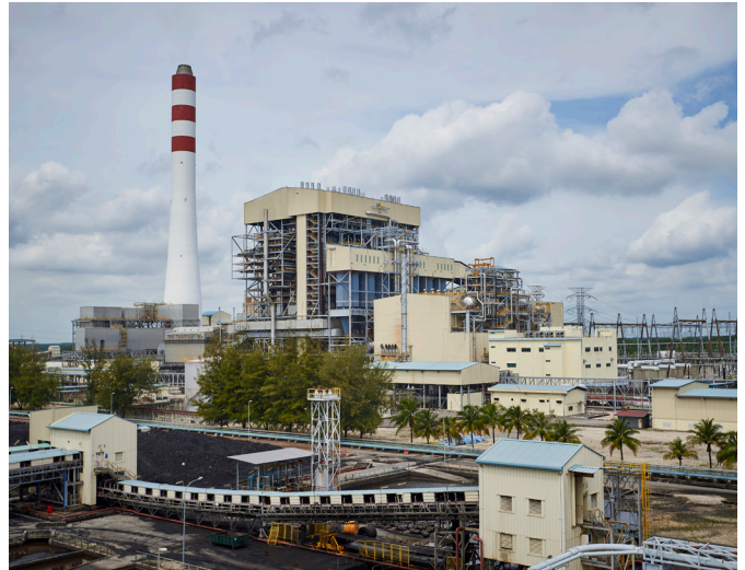
Tanjung Bin Energy Power Plant, Johor
