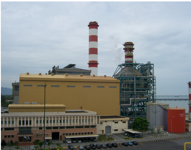
Prai Power Plant, Penang
