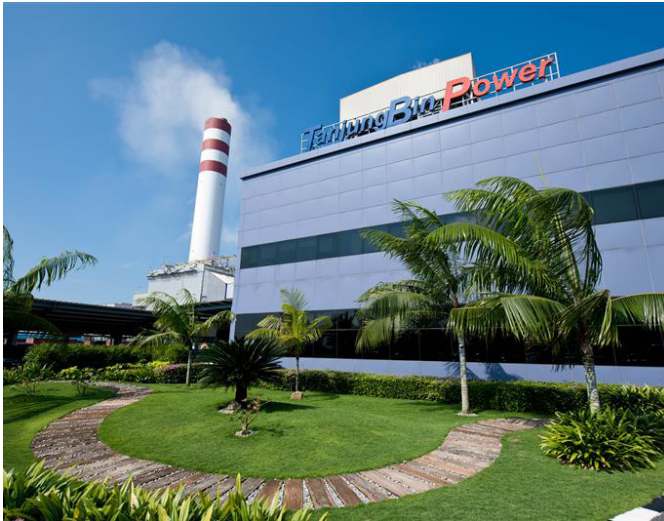
Tanjung Bin Power Plant, Johor
